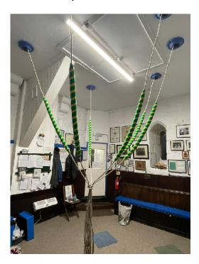
The ropes for bells 1,2 and 3 are 50 foot long, and those for 4,5 and 6 are 53 foot long (yes we do still order in 'old, measurements!) They reach from the folded double tail end, which we hold, in the ringing chamber, through wooden channels in the clock chamber and into the bell chamber, where they go round the bell wheel and fasten in a very secure and traditional way to the wheel cross braces . (see photo of the bell chamber).
